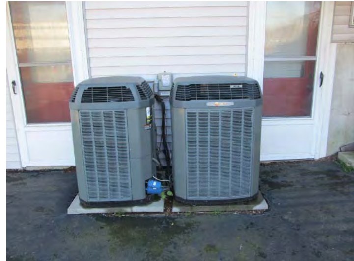
Individual, exterior-mounted, condensers for unit HVAC (heat pump) systems
