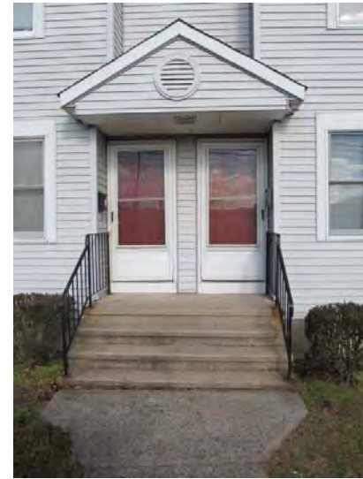
Typical unit entry and storm doors and pre-cast concrete stairs
