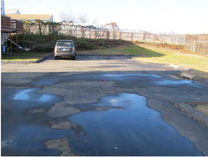
Original asphalt paving at driveway and parking area is in fair to good condition for its age
