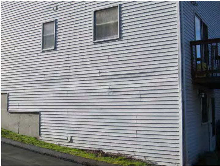
Vinyl siding exhibits isolated areas of minor undulation
