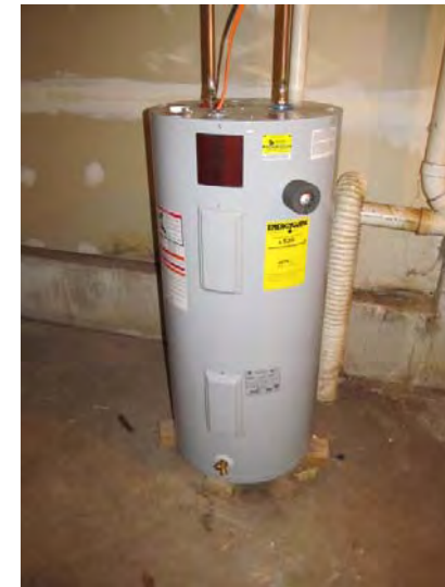
Individual, electric-type, tanks provide domestic hot water at each unit
