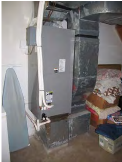
Typical interior-mounted air handler for unit HVAC (heat pump) systems
