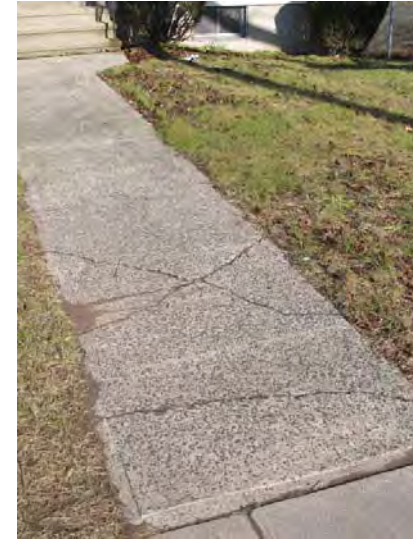
Concrete walkways leading to front entries exhibit cracks and damage at some locations
