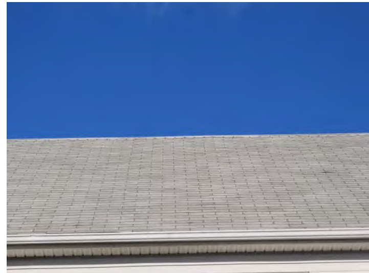
Original roof shingles are in good condition for age but beyond end of typical useful service life
