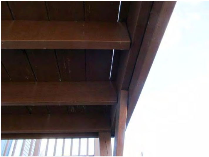
Floor joists at unit balconies/decks lack hangers
